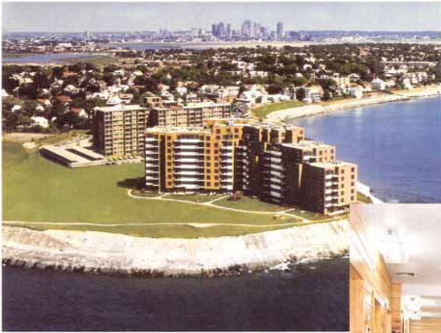
Builder: Sanford Custom Builders. Seal Island, South Boston
